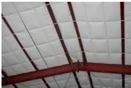
STEEL BANDING Used On Ceiling
