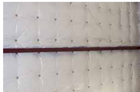
STICK PINS Used On Roof or Walls
