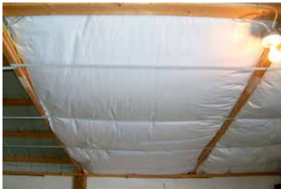
STEEL BANDING Used On Ceiling
