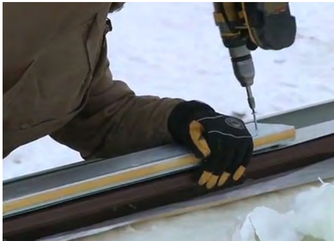
Image showing building without heat loss with Thermal Spacing Blocks installed.
