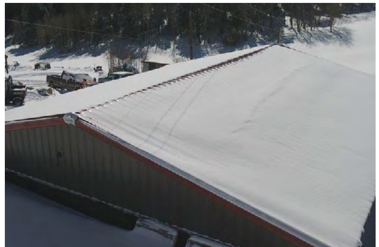
Image showing building without heat loss with Thermal Spacing Blocks installed.
