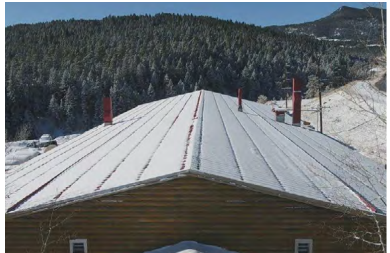
Image showing building heat loss without Thermal Spacing Blocks installed.
